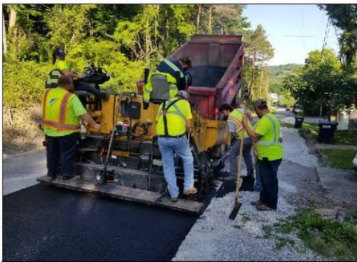
CR 61—County Forces Spot Paving
