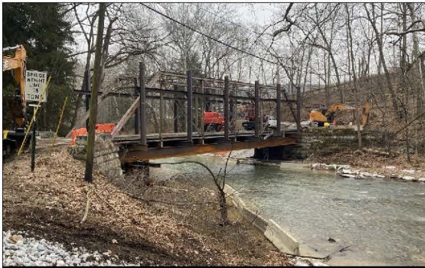
Knox Township Road 289—Historic Truss Bridge Rehabilitation
