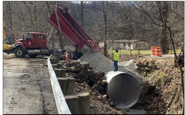
Cross Creek Township Road 173—Bridge Replacement
