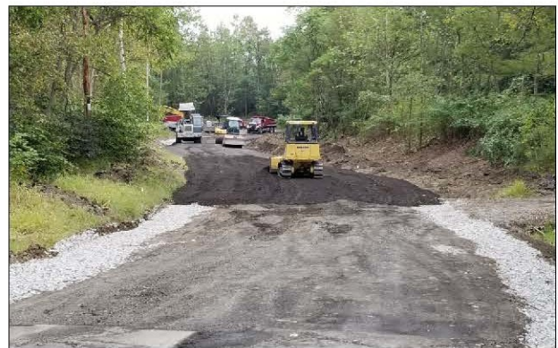
County Road 51—Flood Prevention Project
