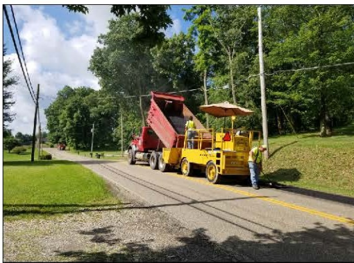
CR 10—County Forces Pavement Repairs
