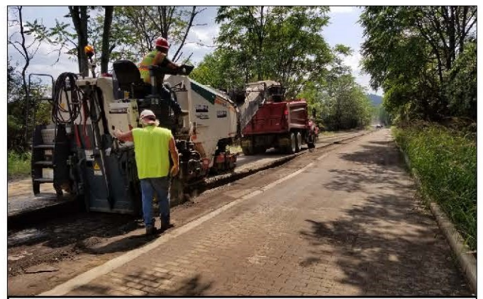
County Road 7C—Exposing brick road with milling machine
