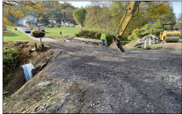
Steubenville Township Road 1235—Emery St—Bridge Replacement
