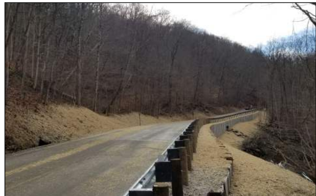
County Road 26 Slip—Repairs Completed
