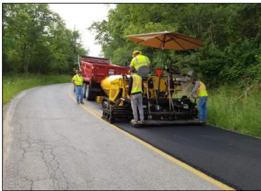
CR 75—County Forces Spot Paving
