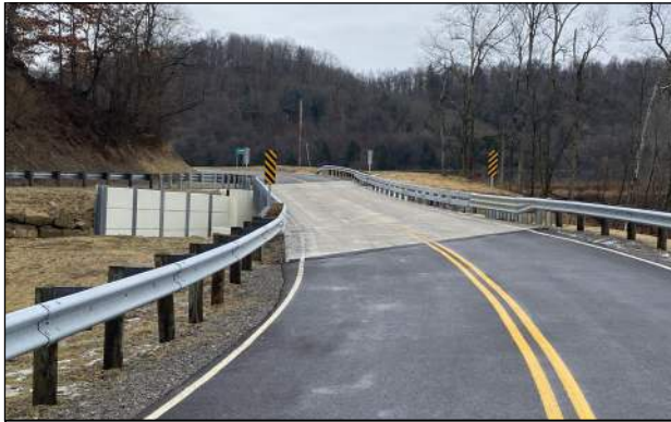
County Road 49—Elkhorn Road—Bridge Replacement
