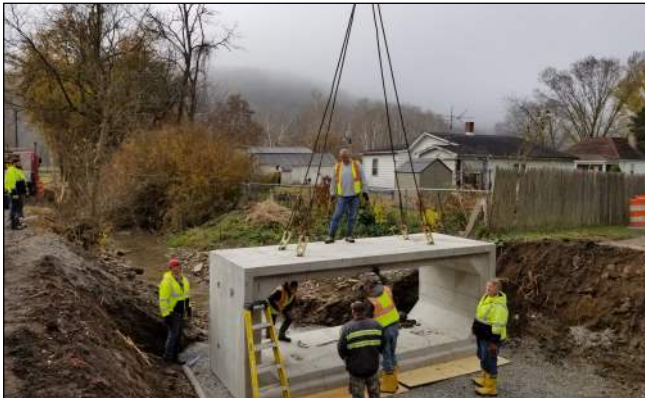
Warren Township Road 1269 Bridge Replacement by County Forces
