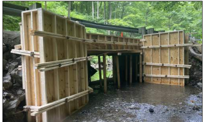
CR 77 Bridge Slab and Wing Wall Replacement
