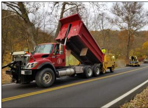
CR 77—County Forces Placing Shoulder Stone
