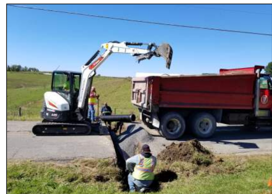
CR 20—County Forces Replacing a Culvert
