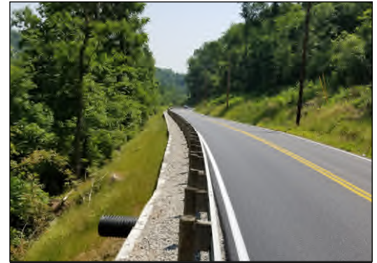
CR 2—Drilled Shaft Retaining Wall and Resurfacing
