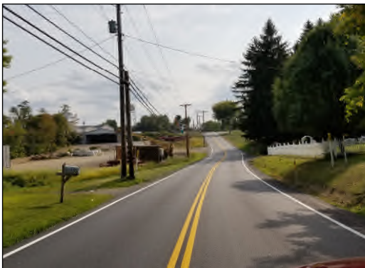
CR 34—Resurfacing with Pavement Markings Complete
