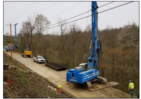
CR 2 —Drilled Shaft Retaining Wall Construction
