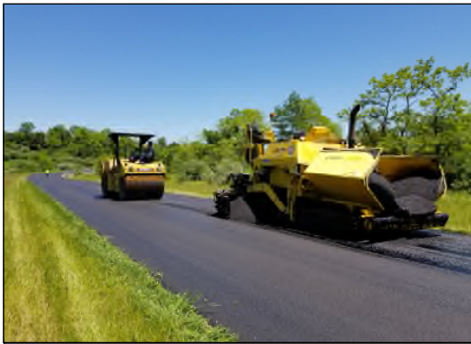
CR 45—Chip Seal Preparation by County Forces
