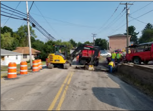
CR 34—Culvert Installation by County Forces
