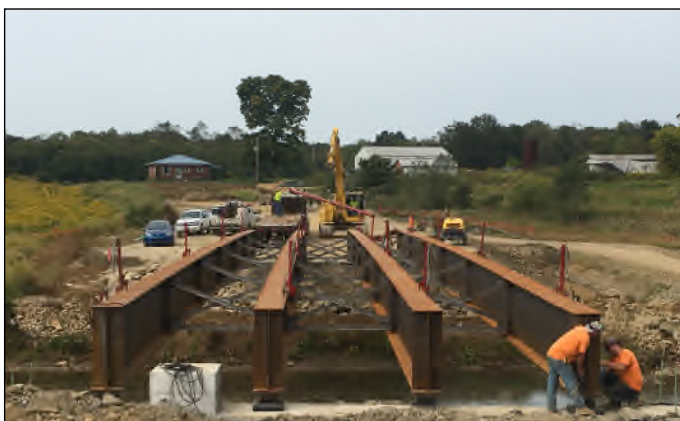
CR 53—Beam Placement
