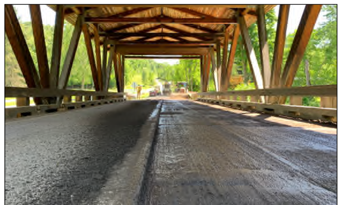
CR 56—Timber Bridge Resurfacing Preparation
