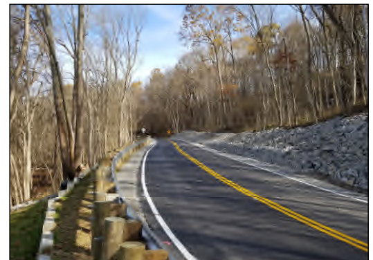
CR 26—Drilled Shaft Retaining Wall Complete
