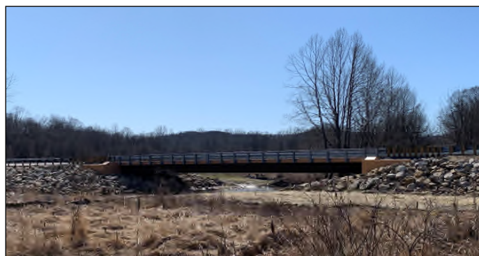
CR 53—Steel Girder Bridge
