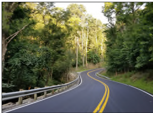
CR 56—Resurfacing with Pavement Markings Complete
