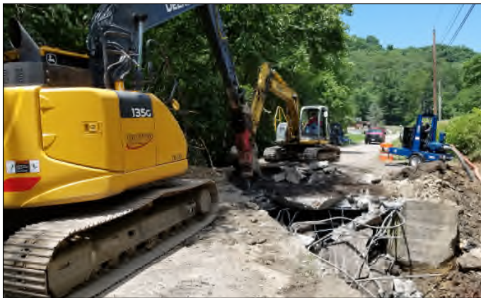
TR 115—Demolition of existing bridge by County Forces
