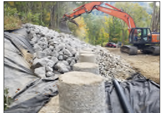
CR 26 —Drilled Shaft Retaining Wall Construction
